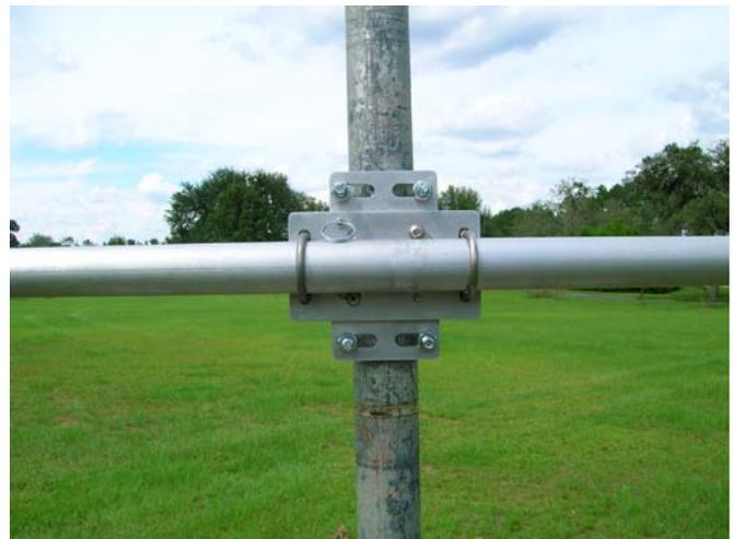
The assembly process can be repeated as necessary to complete your portable or temporary antenna system with as many antennas as you require on your mast. An advantage of the QDAM is the once the positions have been decided for other antennas on the same mast, higher or lower, the previously installed antenna may be easily removed to allow ease of the next mount’s installation or to reinstall to check the total alignment.
